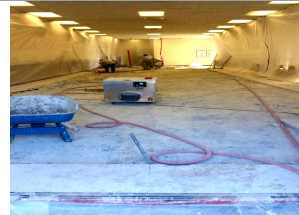
Terrazzo Floor Demolition
